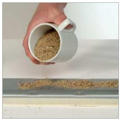
Roughening up the Douche Drain on the outside will ensure sound and solid bonding.
